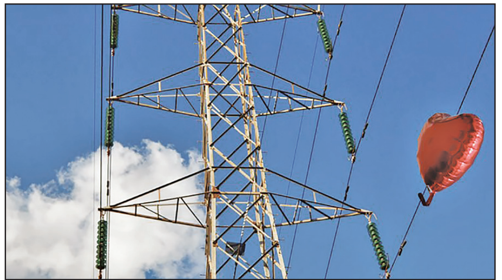
Mylar balloons that have a metallic coating are an increasing cause of power outages in Northern California.
