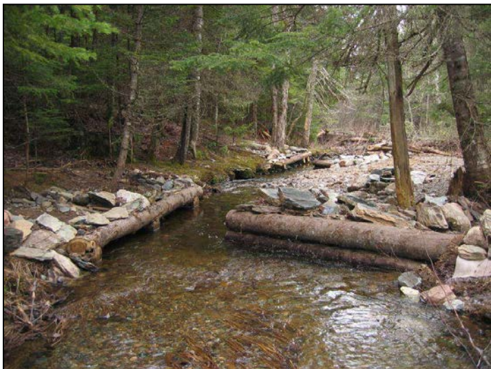
Smith, this workshop. Poster. An example of stream restoration at 5 CDSB Gagetown: a deflector and log cover creates a pool and improves habitat diversity.
