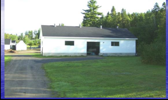
Adult Salmon Holding Building – 6 Tanks and 2 Ponds
