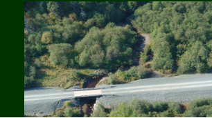
Undersized and perched culverts are replaced with larger culverts or bridges, in-stream habitat is restored, streamside vegetation is maintained or planted and the roads are capped with gravel. This work improves fish passage and habitat, reduces erosion and road flooding.
