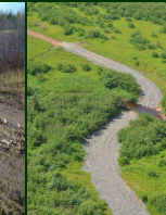
Crushed rock is installed on fords to reduce erosion and sedimentation of watercourses.
