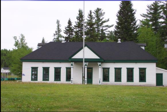
Multi-Use Building – 9 Tanks and Office
