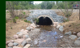
Undersized and perched culverts are replaced with larger culverts or bridges, in-stream habitat is restored, streamside vegetation is maintained or planted and the roads are capped with gravel. This work improves fish passage and habitat, reduces erosion and road flooding.
