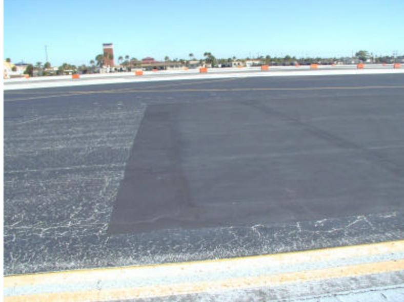
**Figure 4. PCMO surface in October 2012 at MacDill AFB. The adjacent pavement is coal tar that is approximately 14 years old and is severely deteriorated.**
