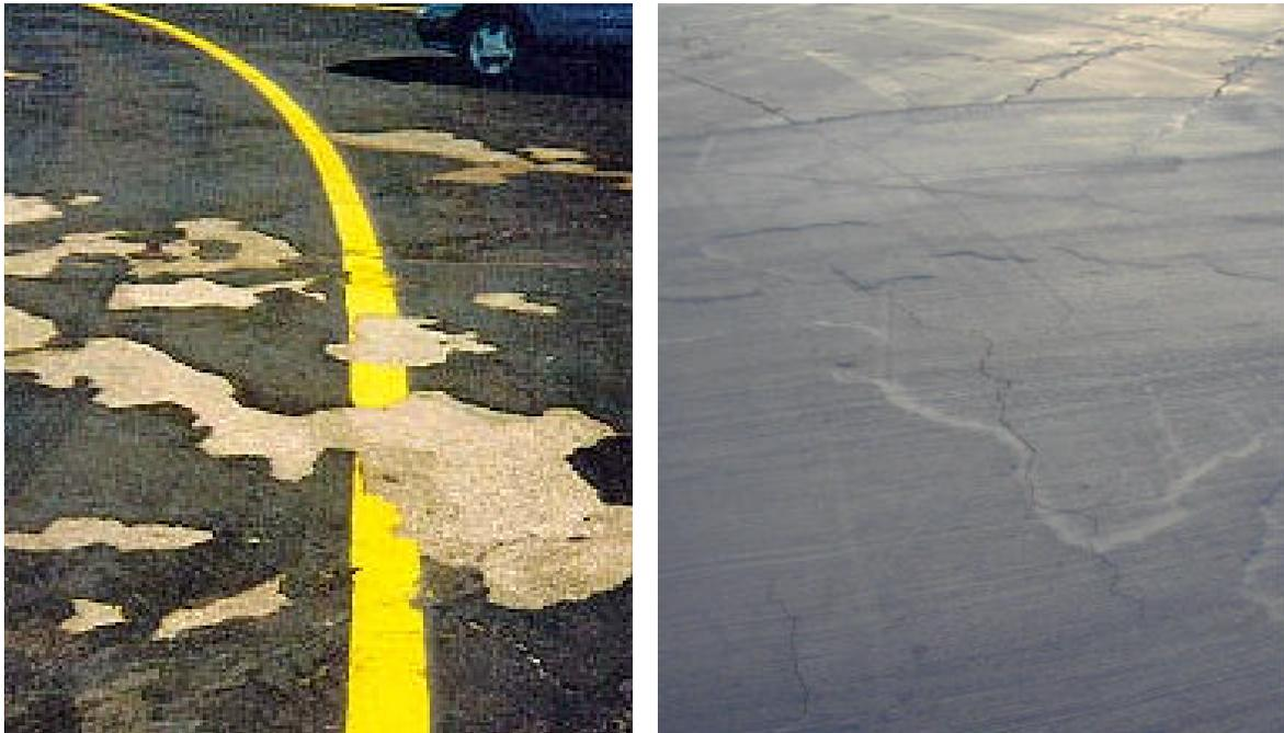
**Figure 7. “Delaminated coal tar area before (2008) and after sealing with PCMO (2012) at Forbes Field, Topeka, KS.**
