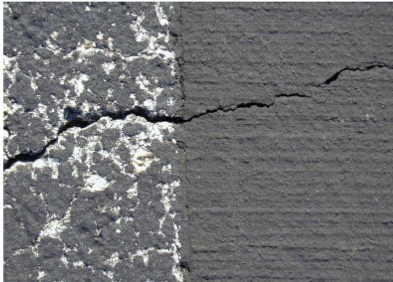
**Figure 5. PCMO section at MacDill AFB showing reflective cracking. Note that the crack has not widened or displayed any raveling from the crack face.**
