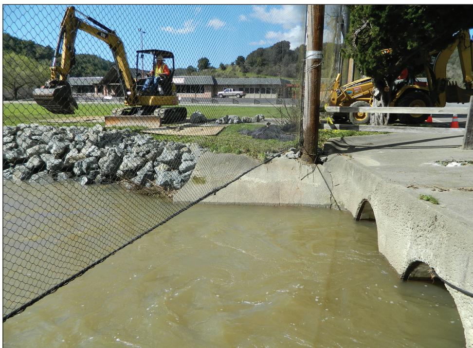
Work crews on Monday were shoring up the bank of San Leandro Creek with heavy boulders at the entrance to Redwood Canyon Golf Course. The creek, swollen by mandatory releases from a bank-full upper reservoir, recently flooded all 18 holes of the golf course.
