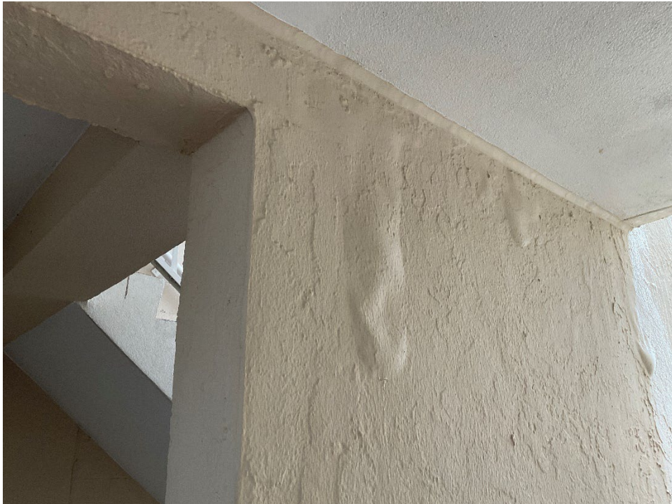
6. Bubbles were observed in the cladding of the exterior near stair towers.
