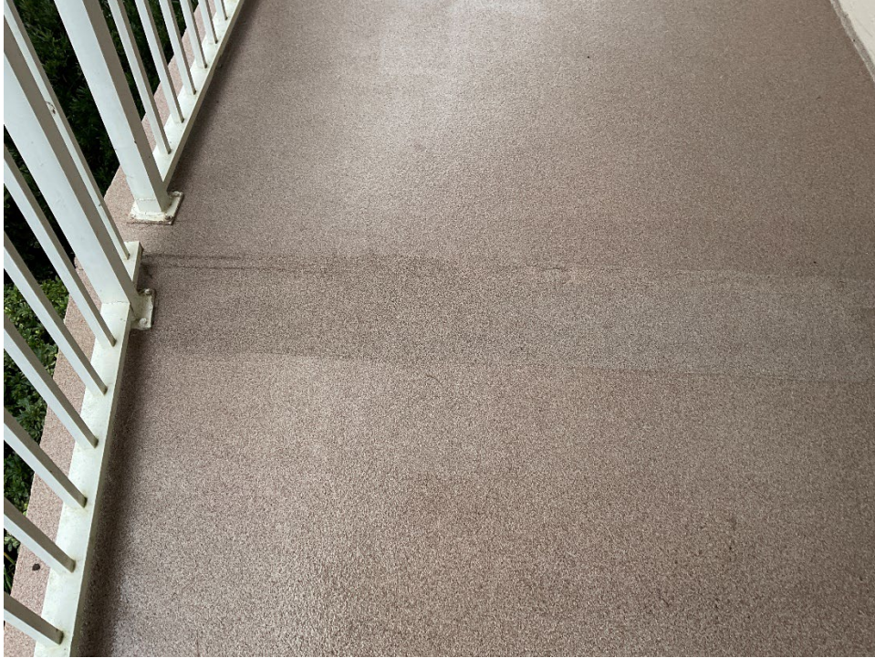
9. View of cracks at an expansion joint in the corridors.
