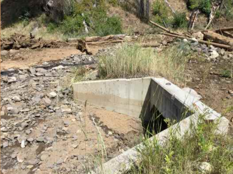
Box culvert on lower Boulder Creek plugged in 2015 and channel carved new path; 2018 work will remove culvert from the floodplain and reshape channel.
