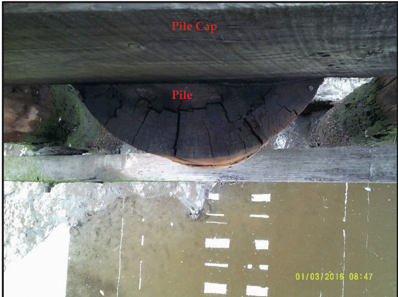
Figure 11. Where the tops of piles are not completely protected by the pile caps, they are susceptible to weather and subsequent wood decay, as viewed from above. The inspection included resistance drilling of a representative sample across the diameter within a few inches of the top surface to detect decay voids.
