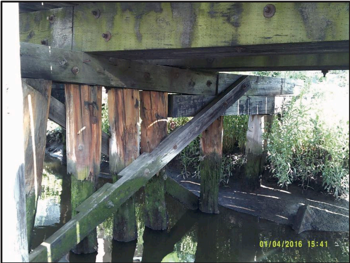
Figure 18. Many of the sway braces are of high-quality wood and are in serviceable condition as is. Should there be a need to repair or replace the piles, the sway braces should be replaced in-kind. Note the extension of the bent, perhaps to carry a switch and second set of rails.
