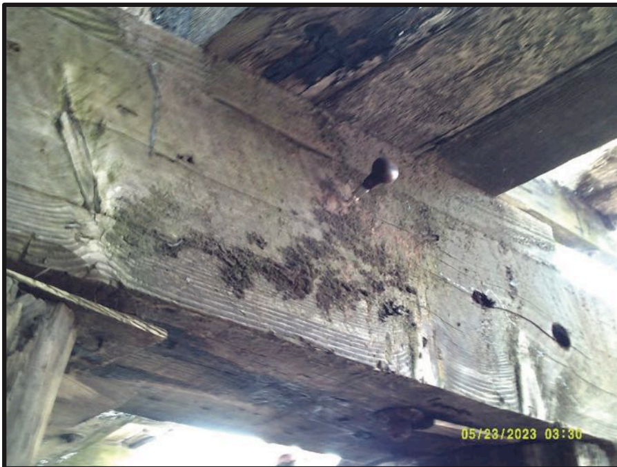
Figure 13. Of the 35 pile caps we were able to inspect, we found nine that effectively have no surviving cross section in at least one location along the length and likely require replacement in kind, pending engineering review of wood assessment findings.
