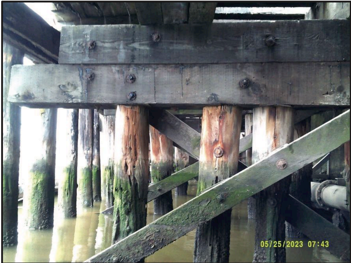
Figure 19. Some of the pile caps are doubled; note the necking down of some piles.
