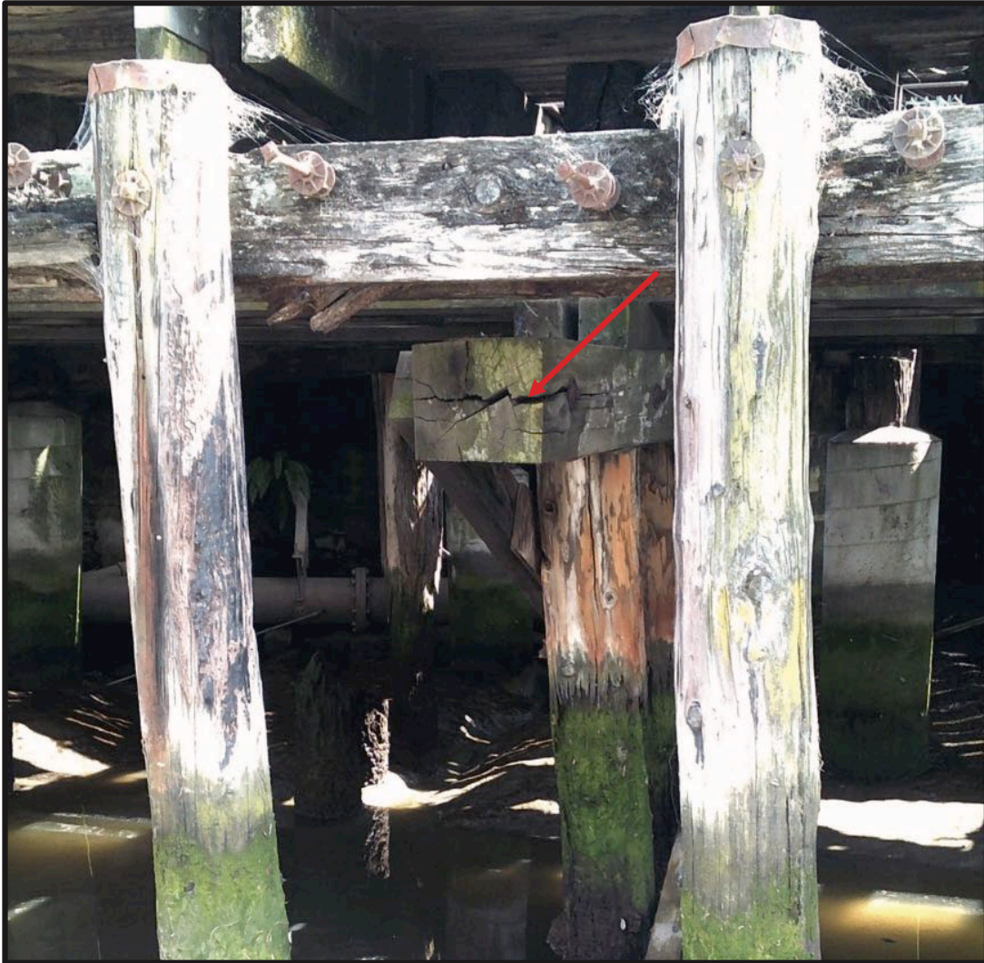
Figure 17. Arrow points to an end split in a pile cap focused on a bolted sway brace – pile cap connection (on the left, or east side, of the cap). The split effectively reduces connection capacity.
