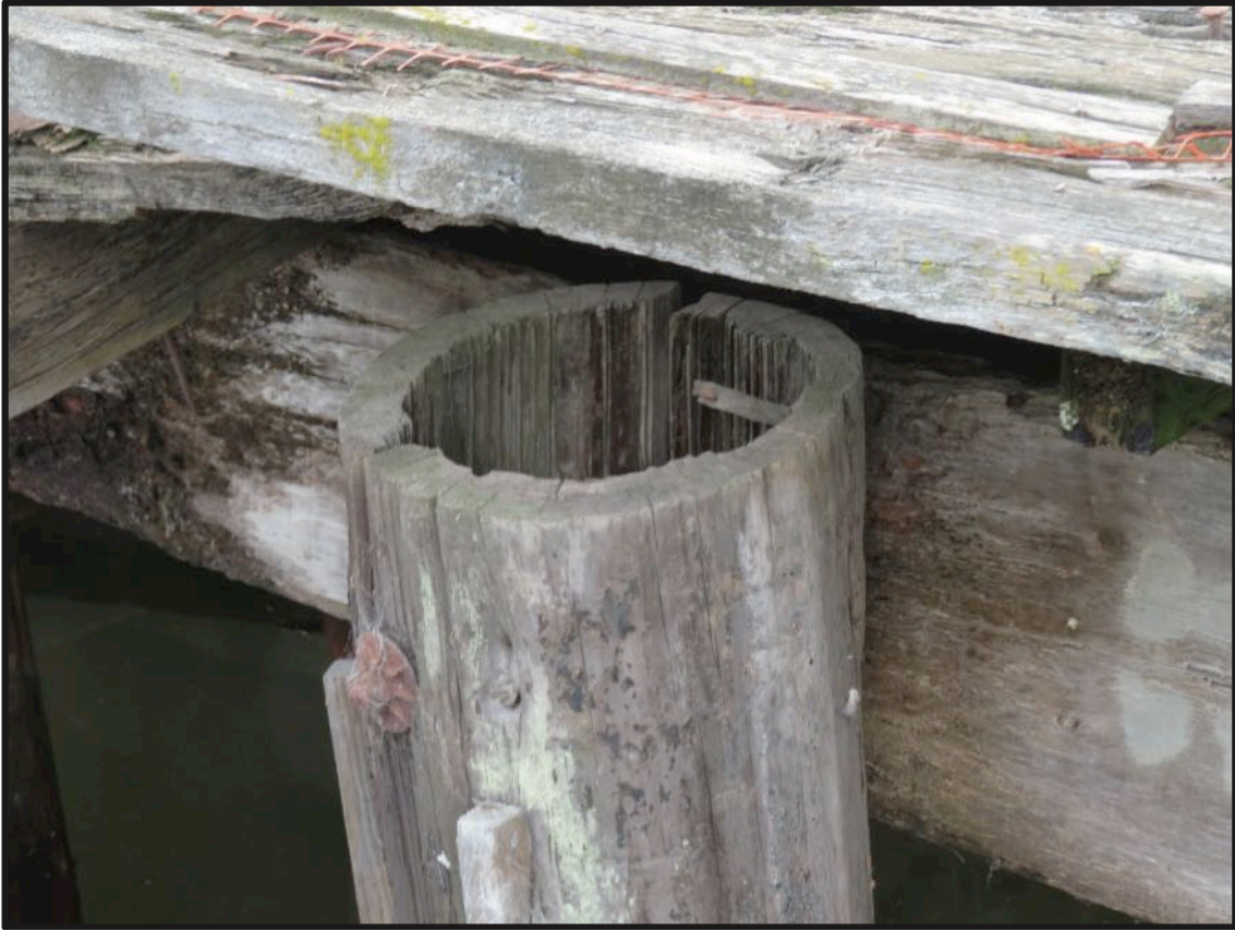
Figure 16. 'Stovepipe' condition in a fender pile; a condition where the wood on the pile interior has decayed, leaving only a shell, typically at the top of the pile. We encountered this condition in the piles that were subjected to resistance drilling in a single instance only.
