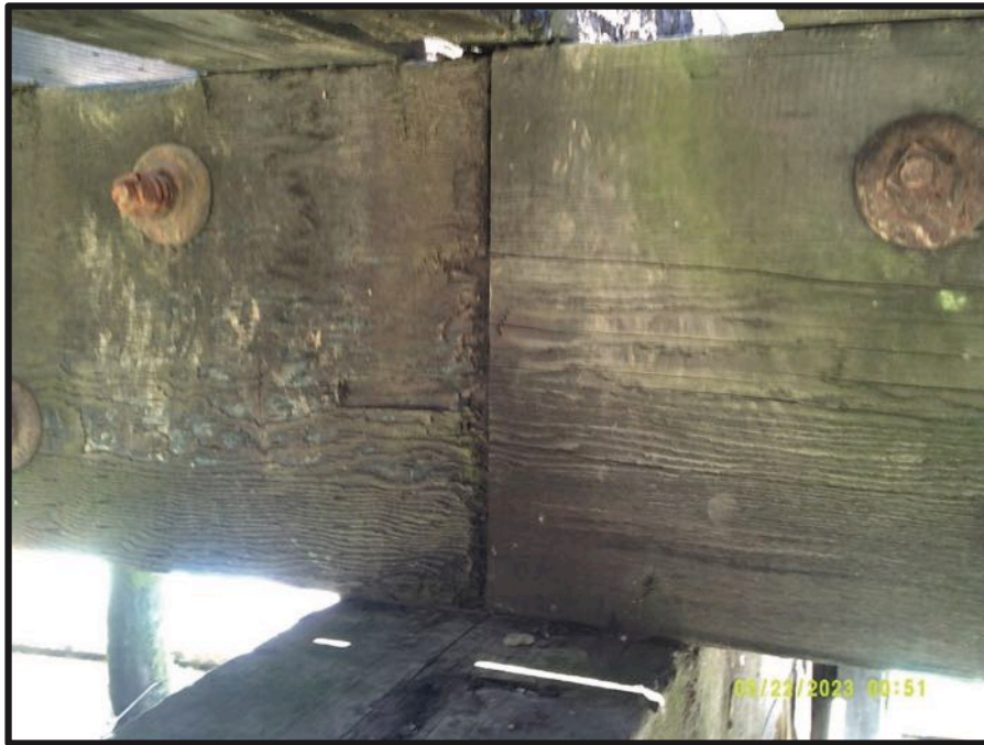
Figure 12. Stringers are nominally 8 x 18, are arranged in sets of three stringers under each rail, and meet over pile caps.
