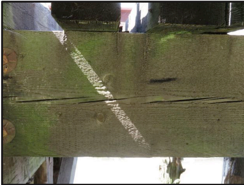
Figure 7. Slope of grain, as indicated by the angle of the seasoning checks, was used to determine the structural grade of this stringer. Seasoning checks are a natural characteristic of lumber and timber and do not affect the strength of the member.
