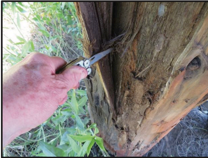
Figure 4. Using a knife to probe the shell of a pile with loose wood fibers to determine the extent of surface deterioration.
