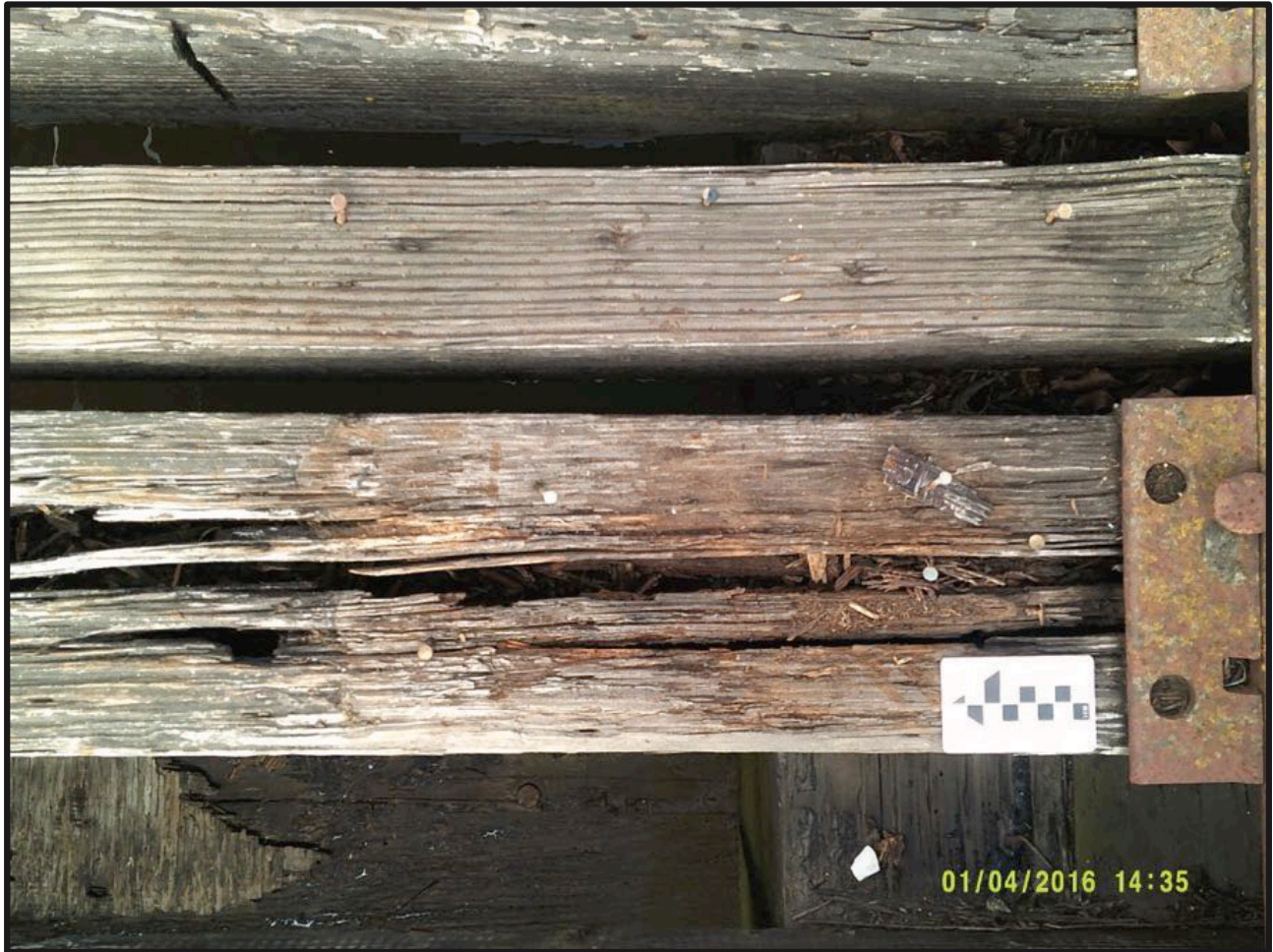
Figure 14. Approximately 23% of the ties have large internal decay voids, many of them accompanied by prominent drying checks on the top surface, along with holes left by spikes that seem to have accompanied an old switch. If left exposed to the elements, the large checks and holes provide a means of water ingress that can lead to additional decay.
