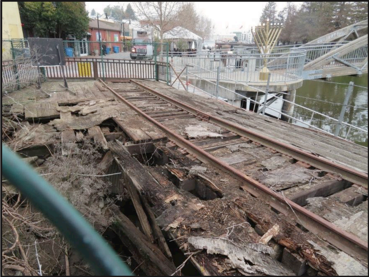
Figure 15. Much of the framing south of the rails is unsalvageable and will require replacement in any repair scenario.
