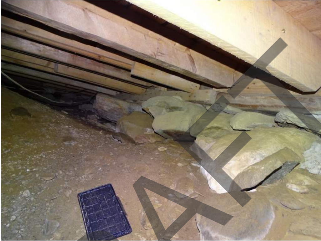
LOWER FLOOR FRAMING AND FAILING FOUNDATIONS
