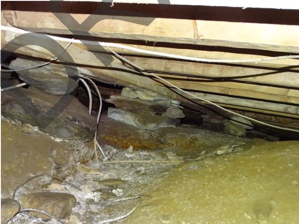
LOWER FLOOR FRAMING AND FAILING PIERS
