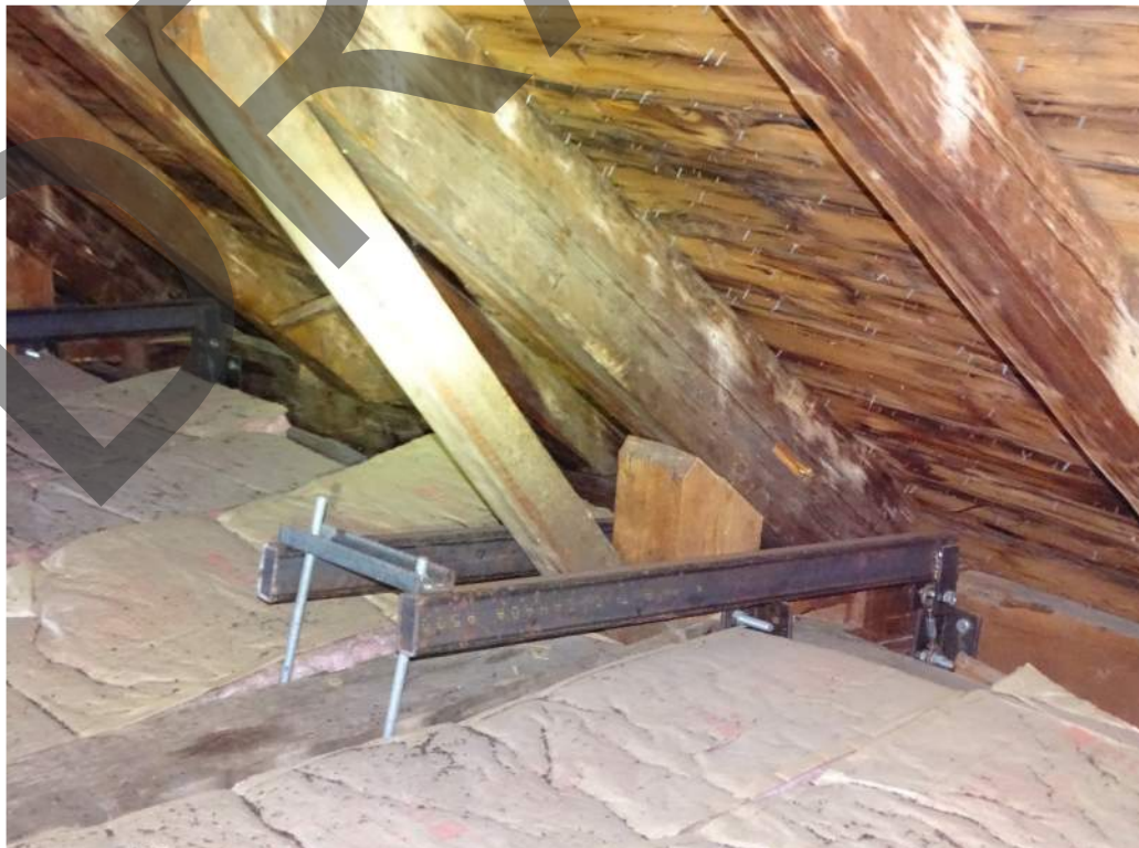
2010 EAVE REPAIR AT TRUSSES
