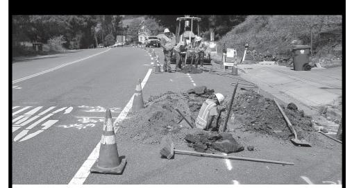
Castro Valley Sanitary District (CVSan) has begun work to replace a forcemain located on Camino Alta Mira and Redwood Rd. The forcemain is being relocated to allow for easier access for maintenance. Terracon Contractors, Inc., have been steadily working on this project and have estimated that work will be complete by mid-June.
