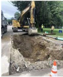
By June 25, 2023, work began on Maple Street installing a new HDPE water main, connections, and manholes. The first new hydrant was installed on July 7, 2023, on Maple Street.
