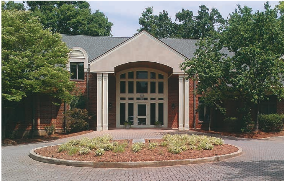
Triangle Arthritis & Rheumatology Associates' new office building in Raleigh.
