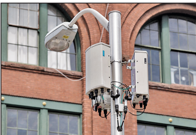
Small cell installations are going up all over the country, paving the way for 5G mobile communication.
