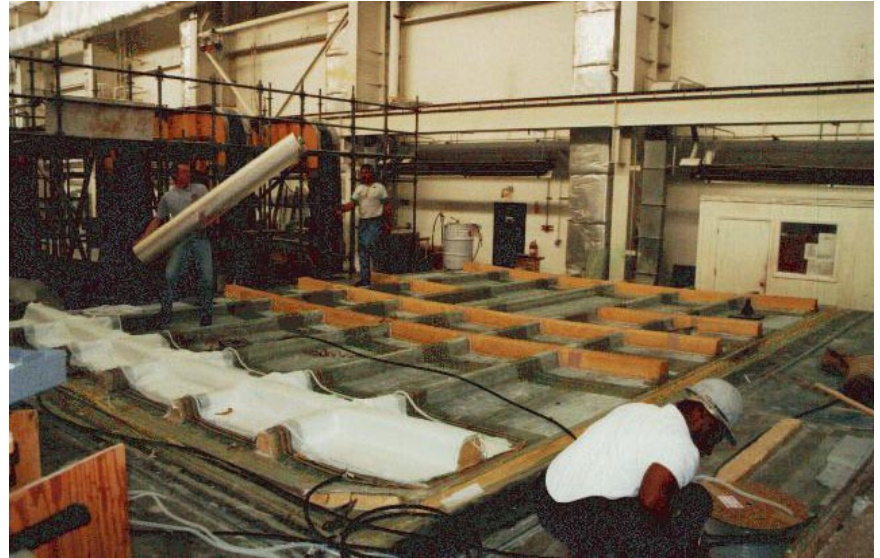
Figure 6 Main deck stiffeners being Infused
