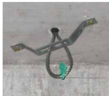
Cable loop installed in a lift head
