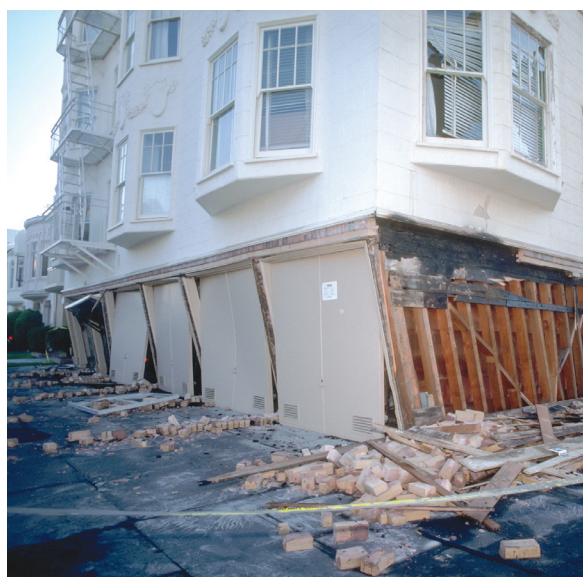
A building in the Marina District at Beach and Divisadero settled onto its buckled garage supports after the 1989 Loma Prieta earthquake.
