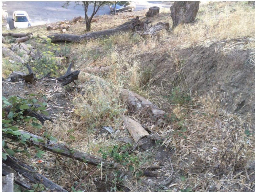
Photo of more hillside with obvious old logs, fencing, leaf buildup and weeds – photo taken 9/6/23
