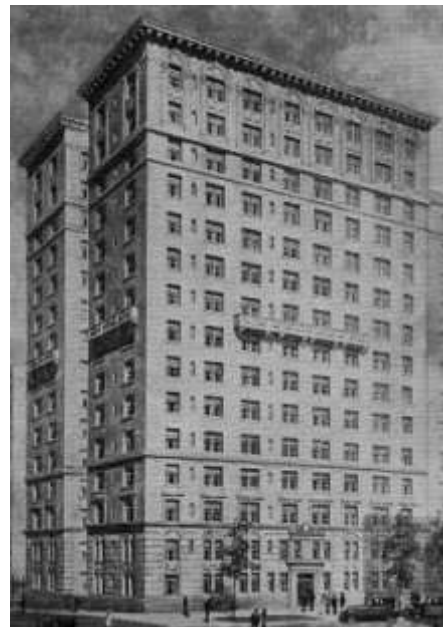
Figure 8. 890-898 West End Avenue (Schwartz & Gross, 1924)
