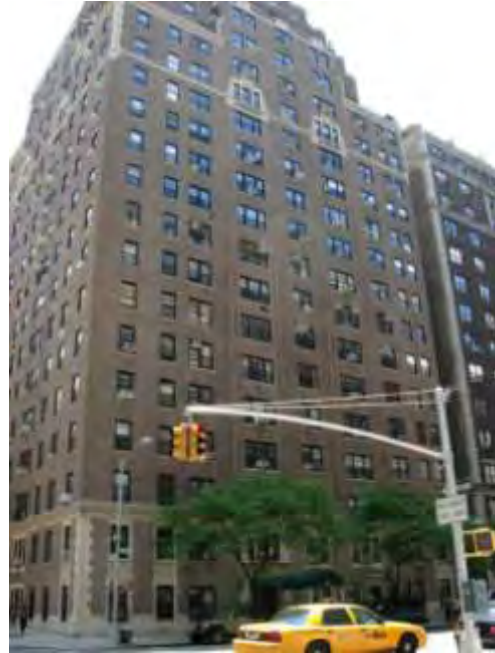
Figure 13. 450 West End Avenue (Boak & Paris, 1930)
