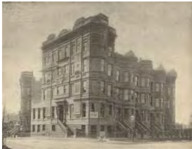
Figure 1. 870-878 West End Avenue (M. V. B. Ferdon, 1891)
