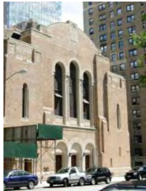
Figure 12. Congregation Ansche Chesed, 824-830 West End Avenue (Edward I. Shire, 1926)
