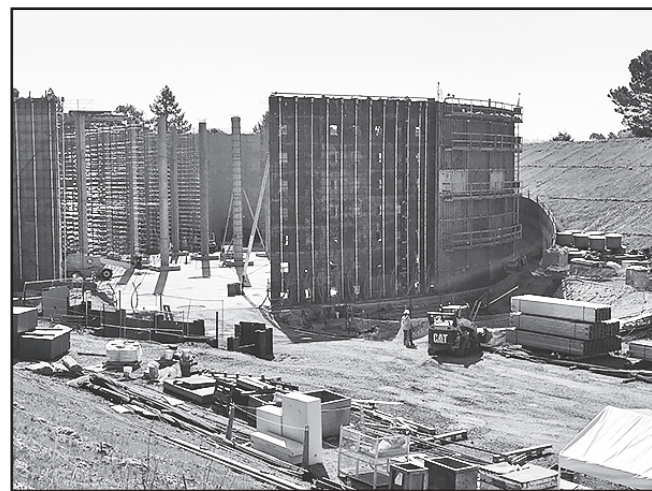
A new 9-million-gallon tank is replacing a reservoir in the Castro Valley/Hayward hills as part of a seismic upgrade being done by EBMUD.
