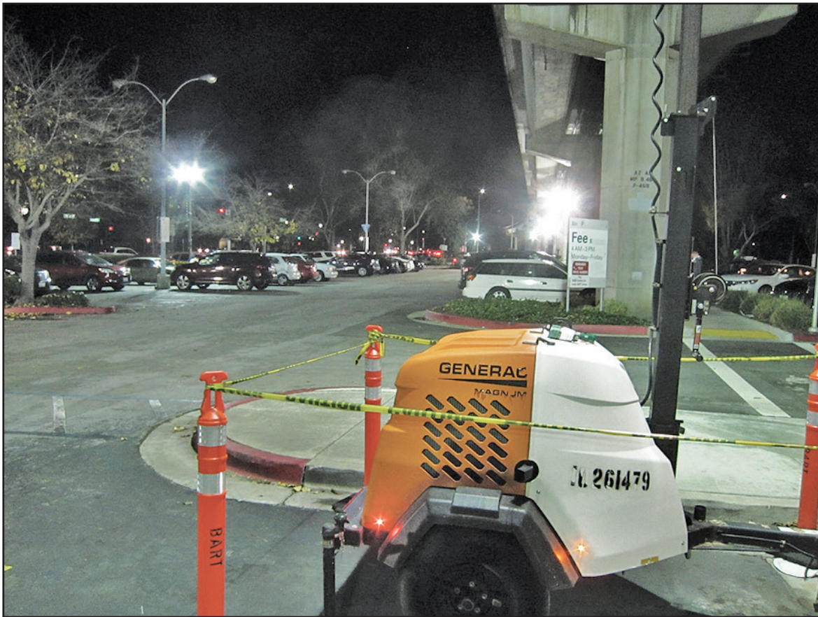
BART installed portable light stands running on diesel generators in the parking lot around the San Leandro BART Station after the parking lot lights lost power when a line was damaged.
