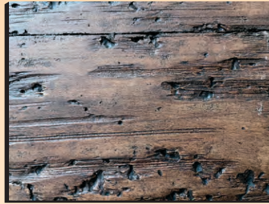
Rustic with or without cracks
