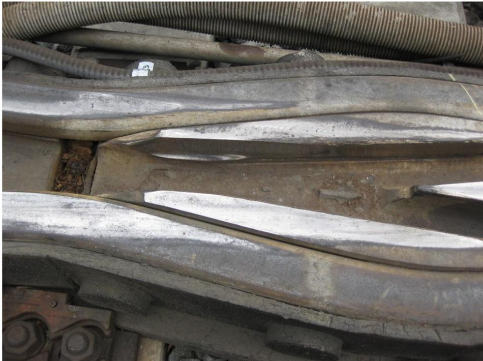
**Figure 7: Observed Wing Rail Wear**
