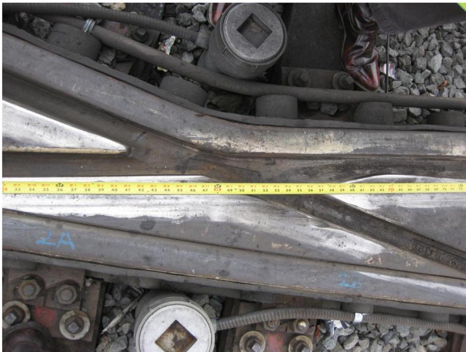
**Figure 8: “Blip” and Ramp on D2**
