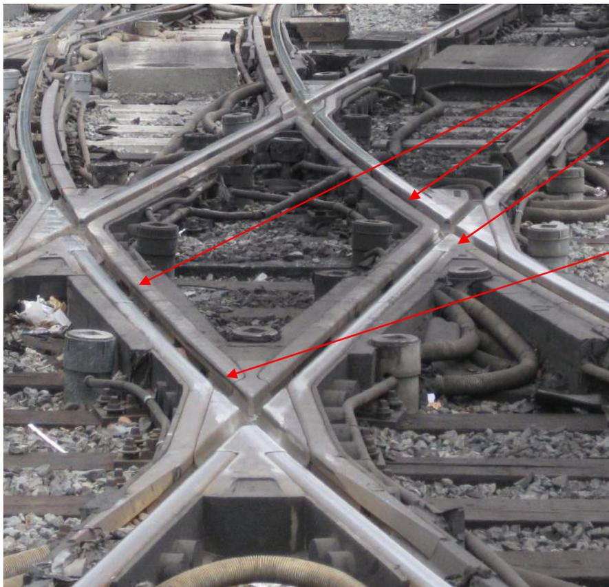
NOTE: With wheels pinching both flangeway guard rails, frog D4 must be struck by passing wheel sets. By observation, both flangeway guard rails are being worn by passing back of flanges.
