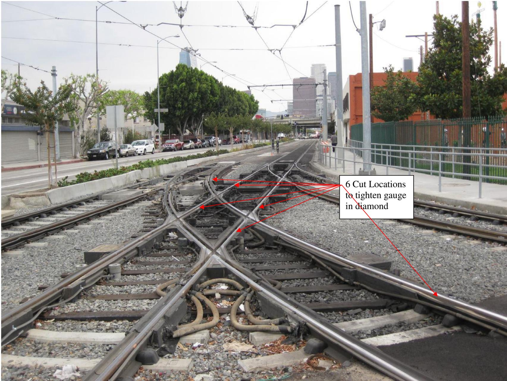
**Figure 14: Locations for Cutting Rail to Restore Gauge**
