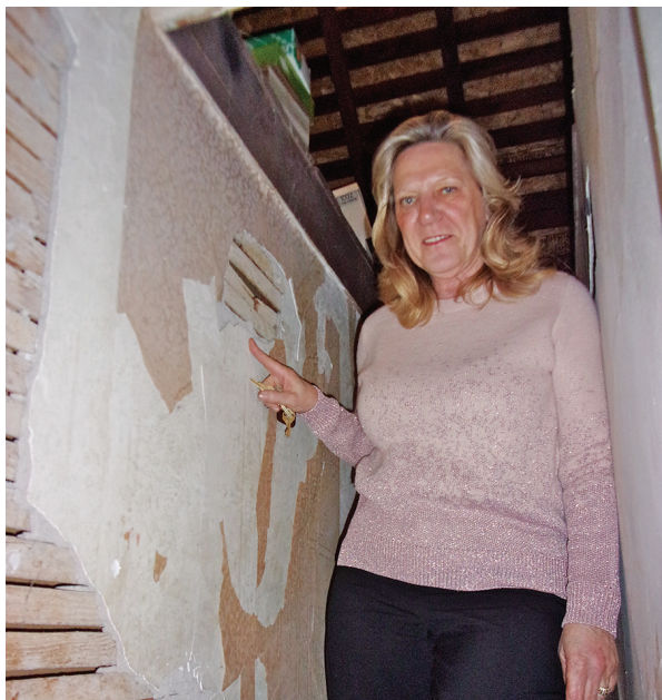
BEFORE: Many layers of lath and plaster walls cover the interior of the Stanton House. This attic entry shows how some portions had fallen away over time.
