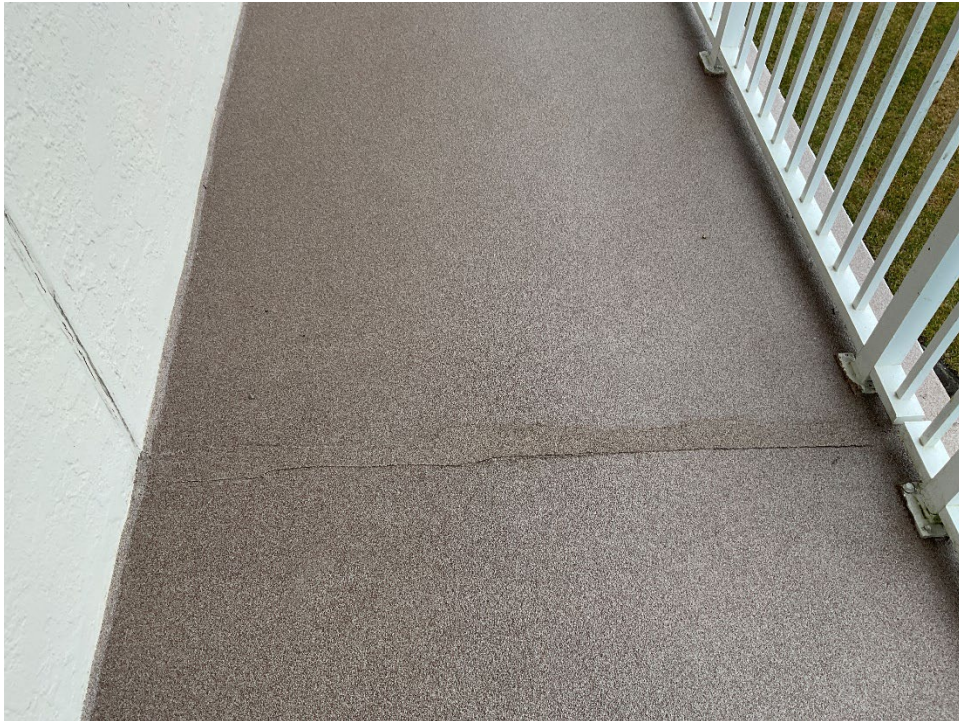
10. View of cracks at an expansion joint in the corridors.
