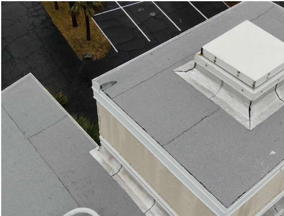
4. We noted an isolated divot in the flat roof section of the equipment penthouse.
